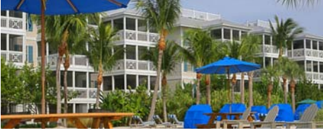
Beach House, A Hyatt Residence Club, Key West, Florida
