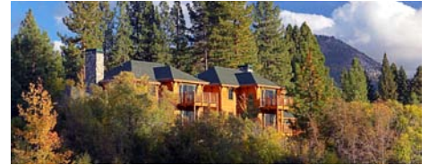
High Sierra Lodge, A Hyatt Residence Club Resort, Incline Village, Nevada
